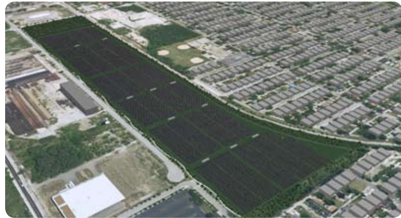
Exelon recently announced plans to operate what will be the largest urban solar installation in the country that, in addition to having a capacity of 10 MW, will reclaim several acres of a brownfield site on Chicago's South Side. Top: site as it looks today. Bottom: Artist rendering of what the site will look like when the installation is complete.
