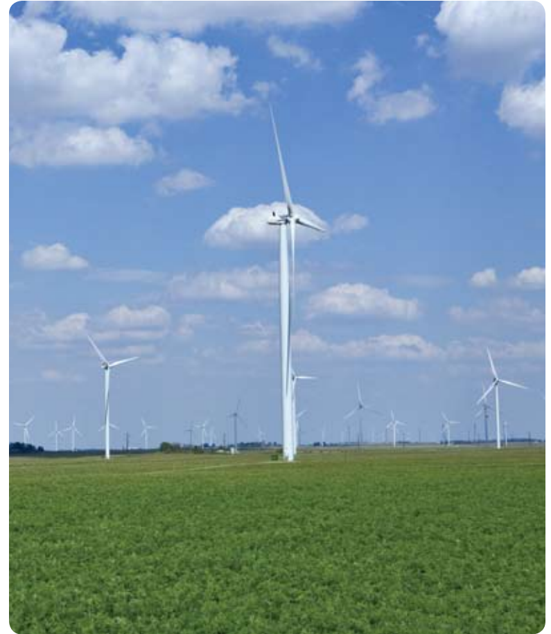
Electricity generated at the Twin Groves wind farm near Bloomington, Ill., is purchased by Exelon Generation.
